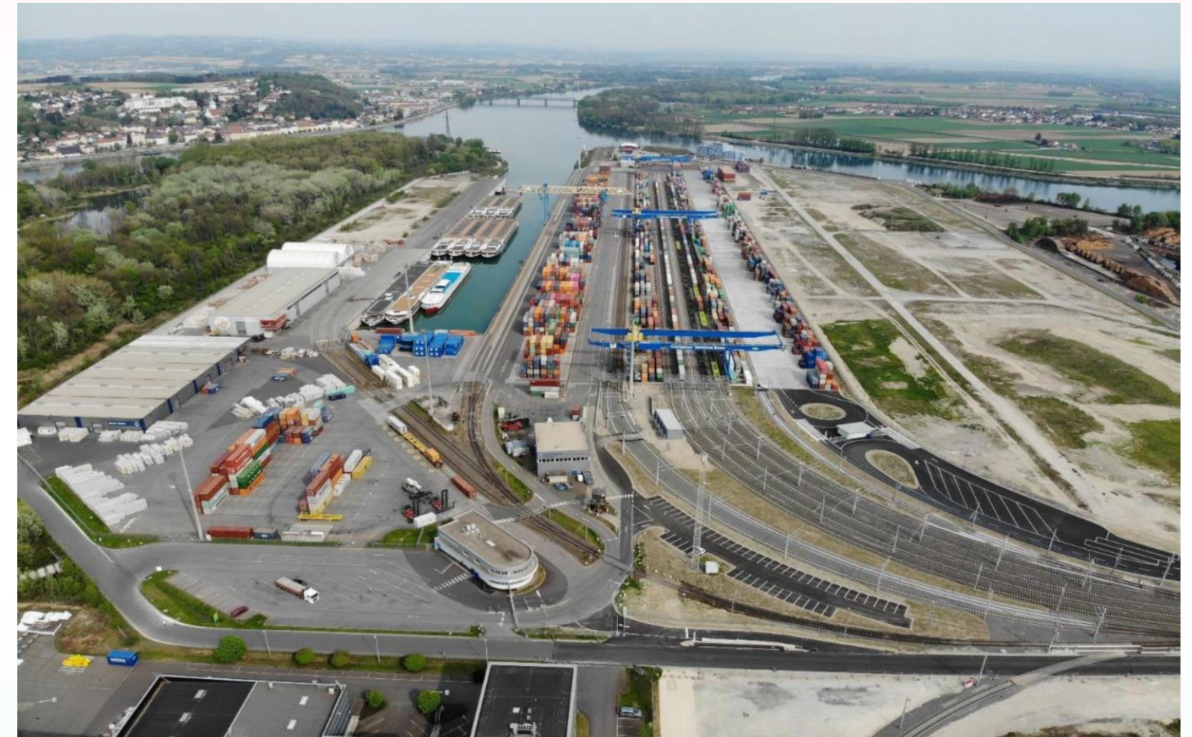
Container Terminal Enns / Ennshafen port (Federal Ministry of Climate Action, Environment, Energy, Mobility, Innovation and Technology, 2021)
