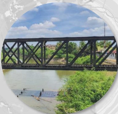
Sungai Golok Bridge across the Kolok River.
